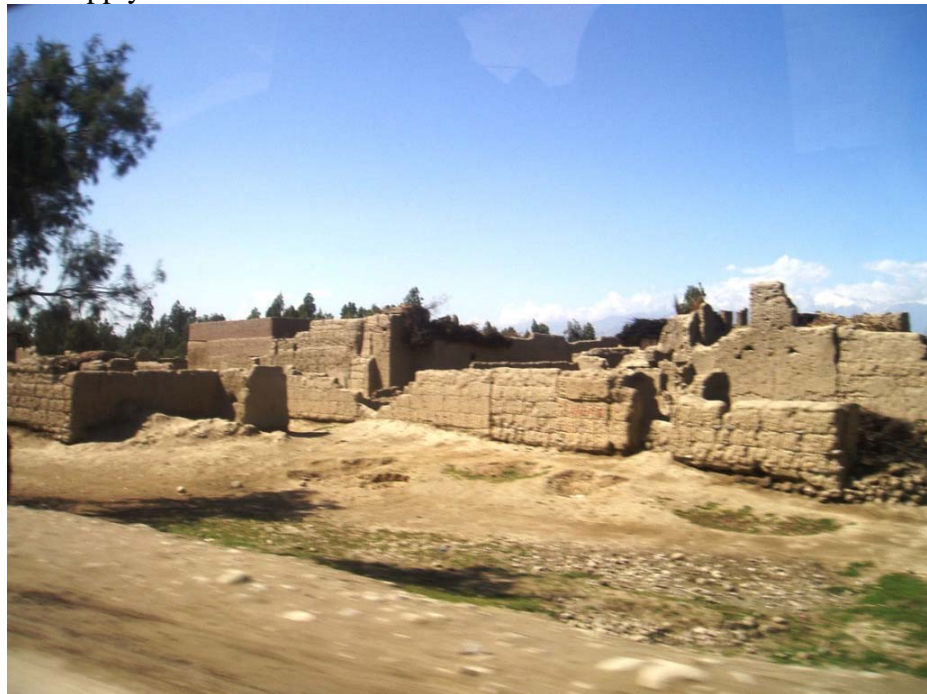
Figure 1: An Abandoned Village Near Jalalabad, Afghanistan
