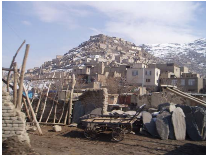
Figure 3: Infrastructure Conditions in Parts of Kabul
