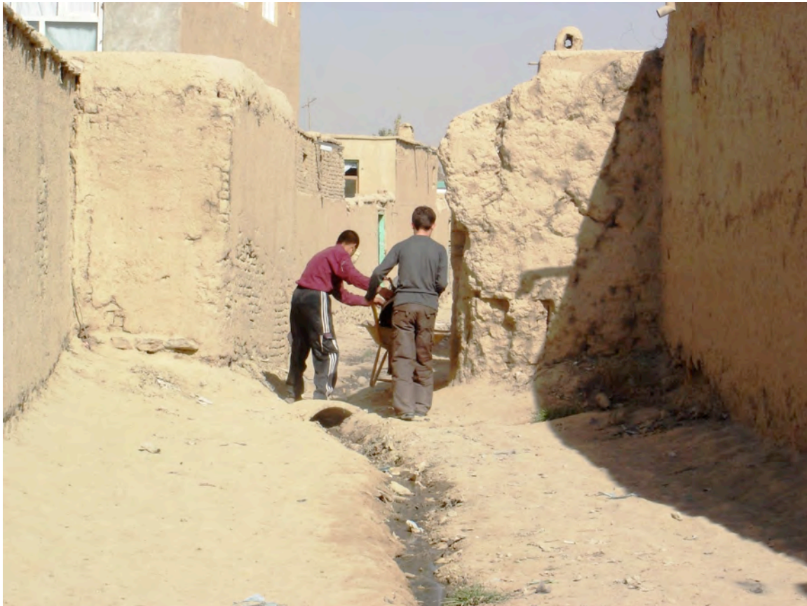
Figure 2: A Passage-Way Before Upgrading
